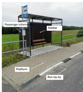
Photo 1. Bus stop with fixtures
