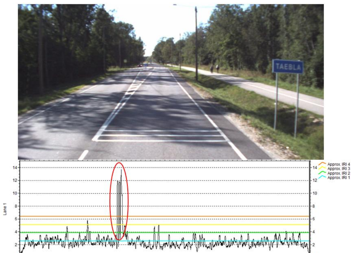
Figure 610_4. Speed bumps in lane 1 at chainage 59000.
