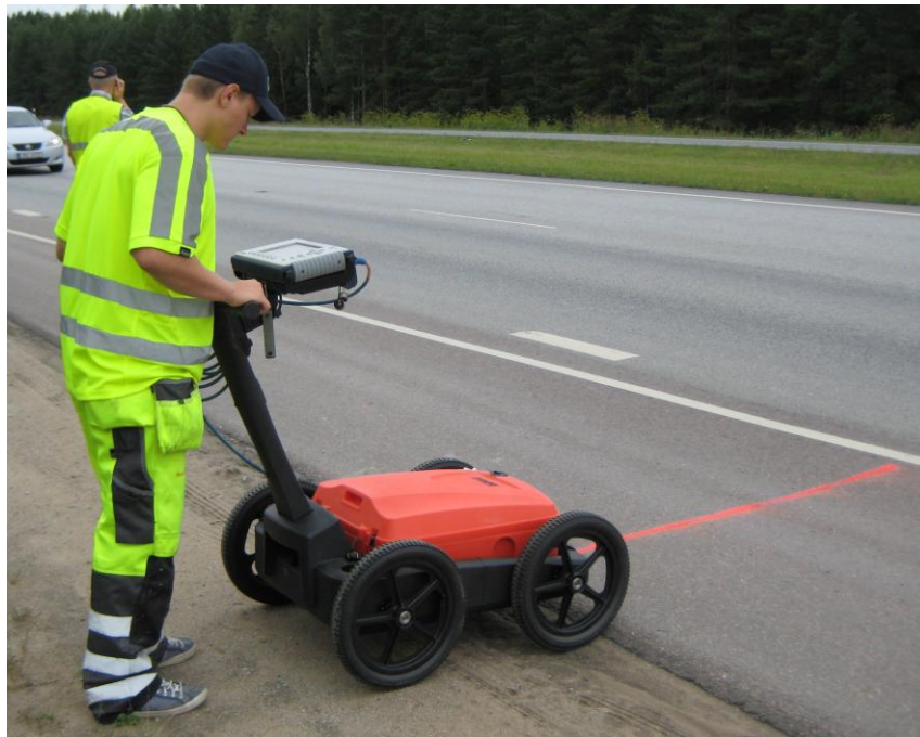
Figure 31_3. The cross-sections were measured with SIR-3000 GPR-equipment.
