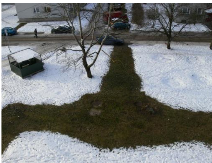
The pipeline heat loss is especially visible in the winter season.
