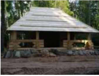
In Võrumaa, the Environmental Inspectorate found an unauthorized building that was raised in the building exclusion zone of a lake. The building is located in the same place, where the owners had displaced their illegally raised sauna as a result of an earlier injunction and fines.
