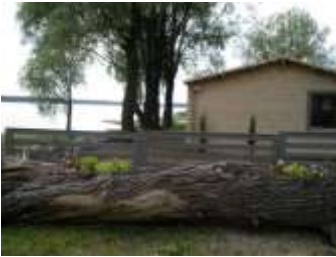
A house constructed in the building exclusion zone of Lake Tamula at the consent of the local government and without decreasing the zone
