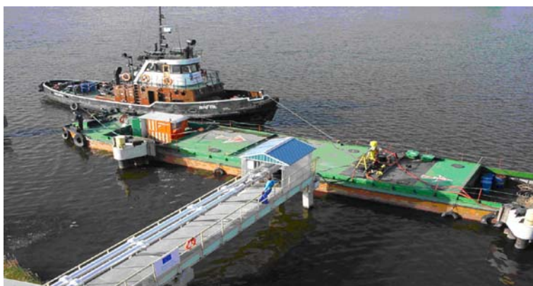
Picture 1. Stationary facilities for bilge water reception at the Ostrów Grabowski in Szczecin (Poland)
